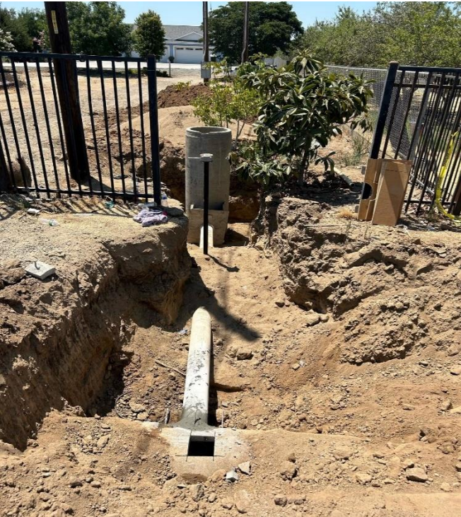
Installed New Turnout for Landowner on the 24.2-9.0 on Road 24 South of Avenue 19
