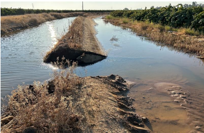
Repaired Sinkhole on the 6.2-16.9 just West of Highway 145 along the South Bank
