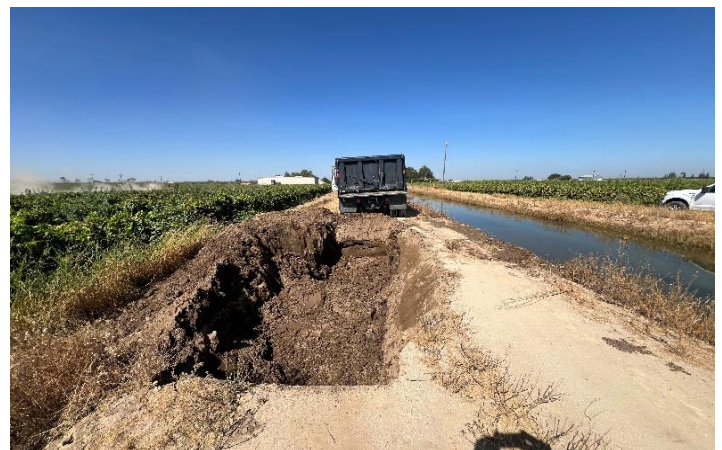
Repaired Sinkhole on the 6.2-16.9 just West of Highway 145 along the South Bank
