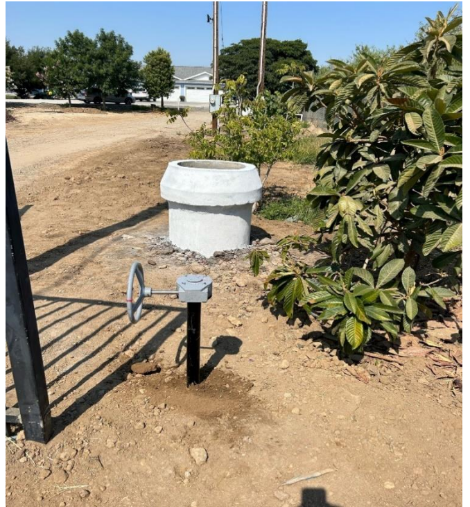
Installed New Turnout for Landowner on the 24.2-9.0 on Road 24 South of Avenue 19
