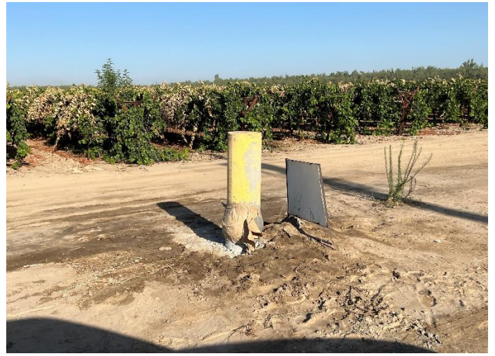
Repaired Leaking Air Vent on the Galeener Pipeline along Road 24
