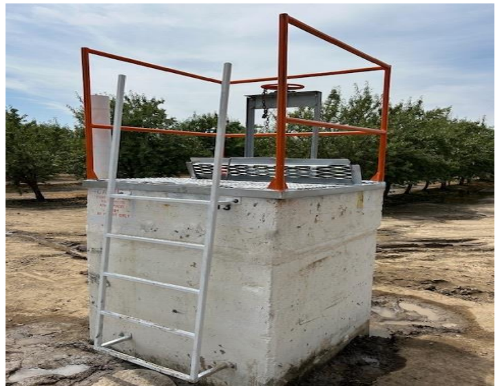
New Safety Railing and Ladder on Clark Pipeline
