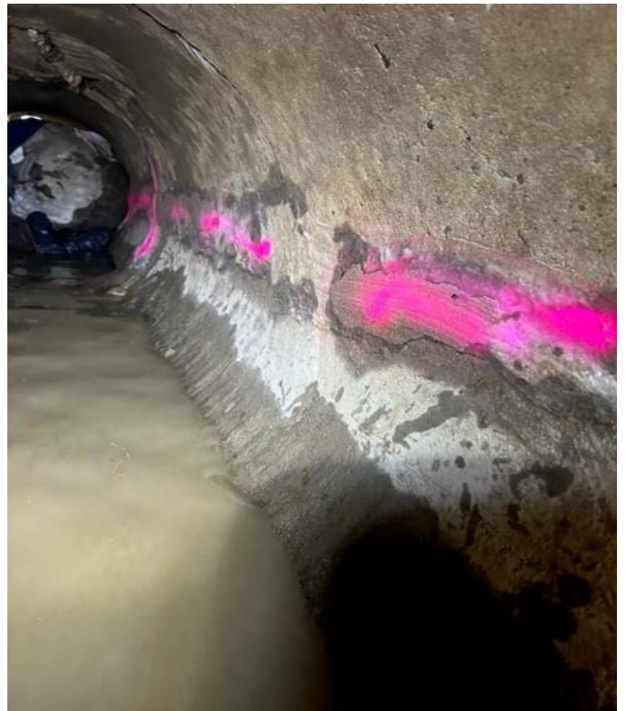
24.2-21.1 West Pipeline on Avenue 11 Showing Parallel Cracks on Pipeline
