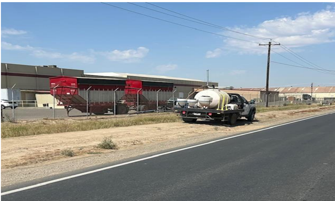
Spray Truck Spraying on Road 26 Schmitz Canal
