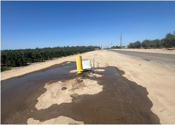
Repaired Leaking Air Vent on the Galeener Pipeline along Road 24
