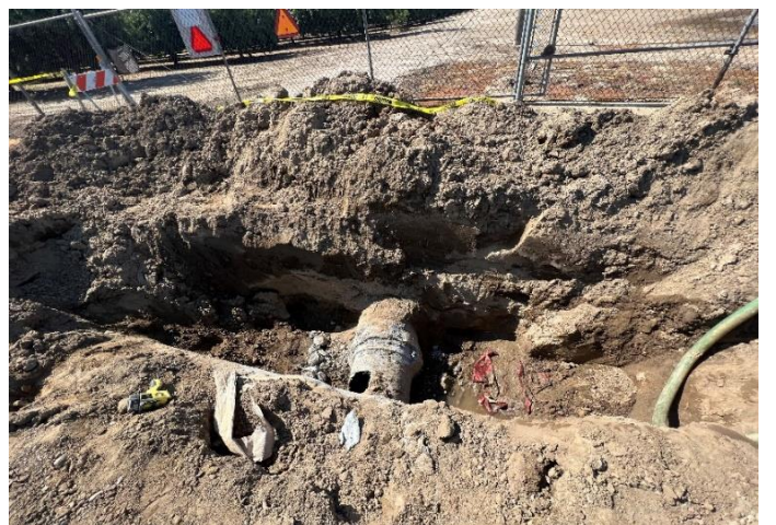
Cody Pipeline Avenue 13/Road 24 (Techite)
