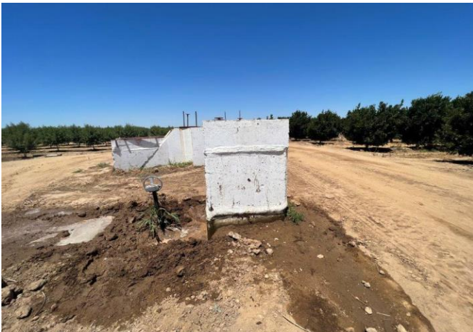
6.2- 14.5 Turnout Leak repaired
